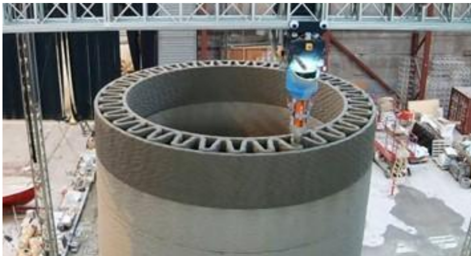
Figure 7: Additive manufacturing of concrete wall via crane (2022) 3D printed wall.jpg[photograph]. Wikimedia Commons. https://upload.wikimedia.org/wikipedia/commons/f/ff/3D printed wall.jpg
