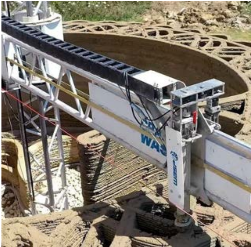
Figure 6: 3D printed clay composite wall structure with internal cavities
