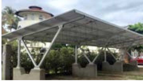
Figure 3: V Carport Design (“The Role of Solar Carports”)
